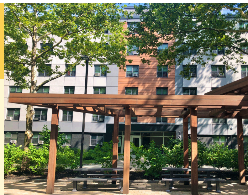
Baychester Houses - Renovated apartments and outdoor spaces
