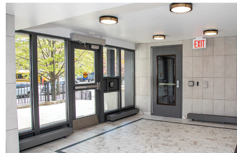
Independence Towers: Renovated lobby
