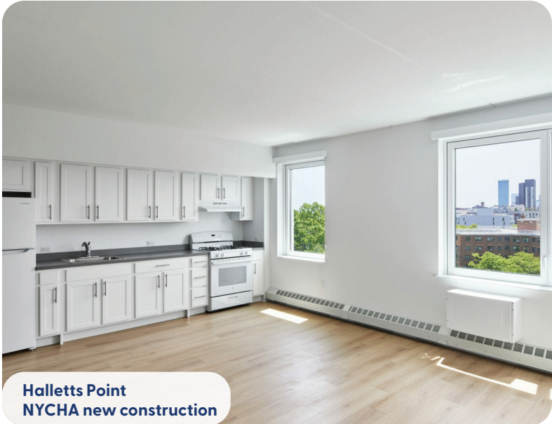
Open layout apartment with resident-controlled HVAC systems
